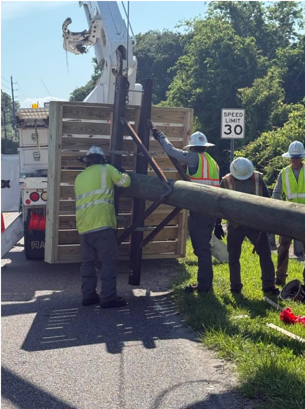
FPU Team attach and brace the platform – Egan's Landing, Simmons Road
