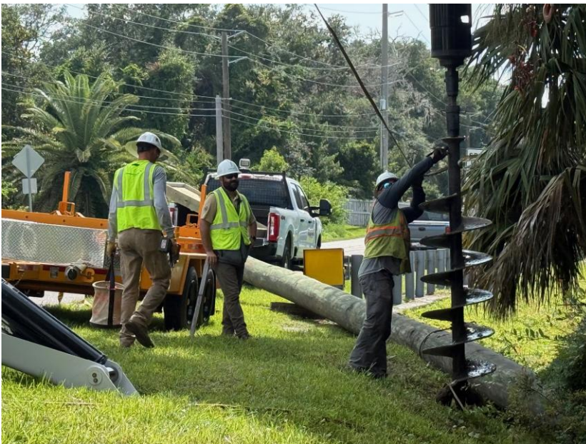
FPU Team drilling the hole – Egan's Landing, Simmons Road
